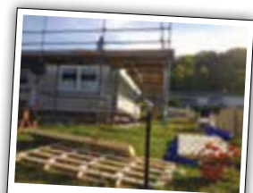
Application of structural insulation board
