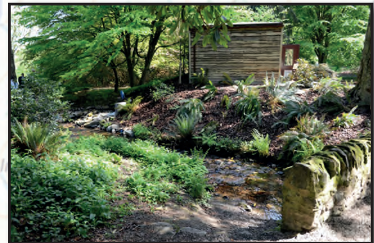
Figure 1 - Powerhouse of a small hydro scheme. Moss covered outfall into the burn seen on the left. Timber clad and sedum roof structure.
